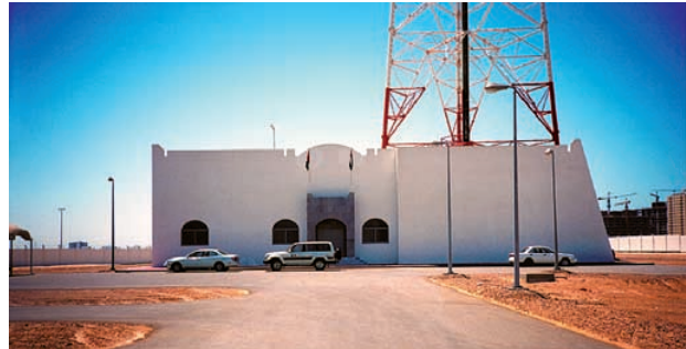
FIG 1 Main building of transmitter station in Dubai
